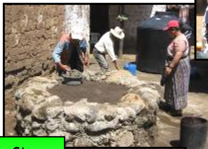
Stone base is prepared for tank to collect rain water.
